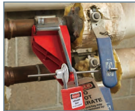
F36-1 Press the butterfly valve handle with a strip compression block F36-2 Press the valve handle with a circular compression block
